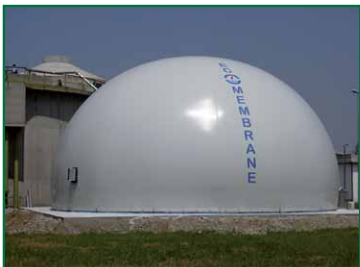
3 membrane biogas holder
